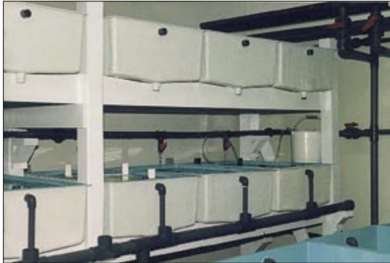
Figure 32: A typical broodstock conditioning system.
